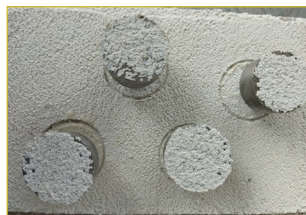
Fig. 3 Cohesive failure of the coating based on Vinnapas EP 3360 Rottura coesiva rivestimento a base di Vinnapas EP 3360
