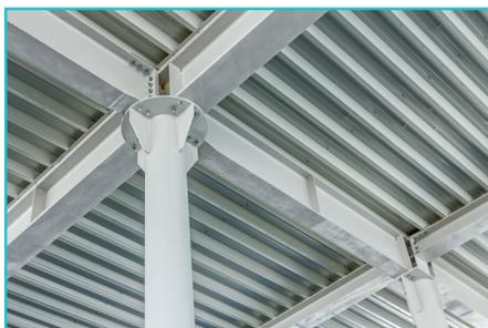
sistance, thus providing vital extra time for evacuation and firefighting efforts. Upon exposure to fire, the paint expands from a thin coating into a thick, flame-resistant foam. This foam then solidifies into a protective char, offering substantial heat insulation to the underlying material.
